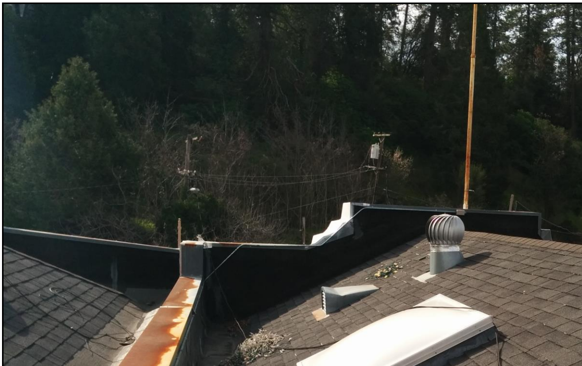
Figure 5: Unbraced roof parapet
