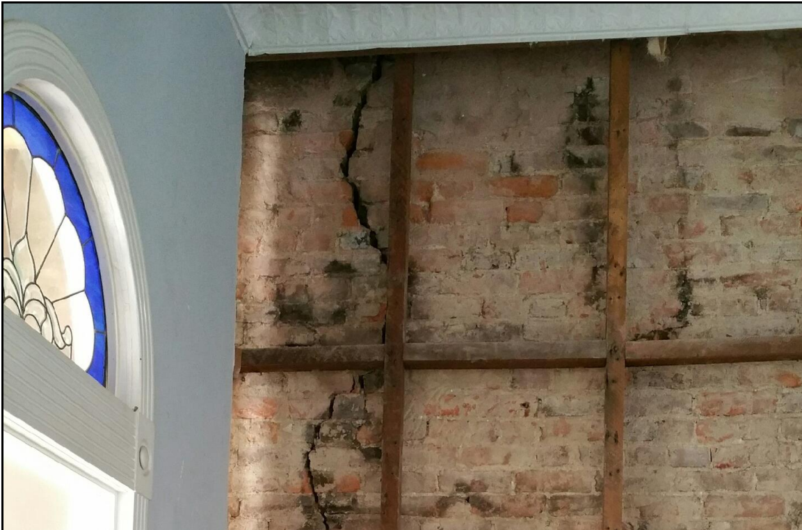
Figure 1: Large cracks in the west masonry wall.
