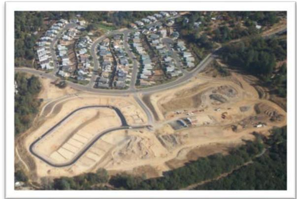
3. In cases where steep slopes will be created, interceptor ditches shall be constructed at the top of slope. These ditches are intended to catch water and reduce potential erosion. To the greatest extent possible, ditches shall be installed in a manner as to be unobtrusive and unnoticeable from the bottoms of the slopes.
