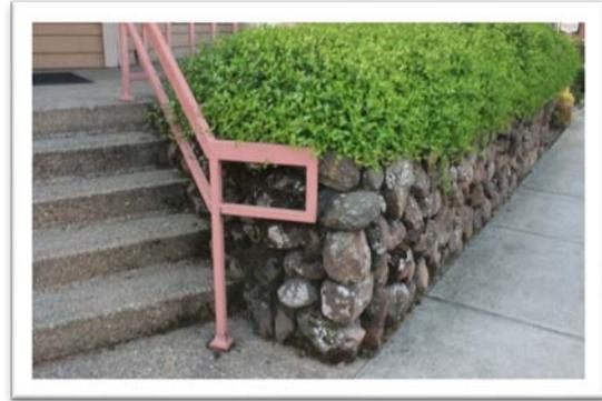
*Where retaining walls are required, these elements should be constructed using natural stone wherever possible.*
