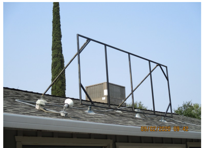
Figure 7 Roof sign support structure and lighting. Staff photo.
