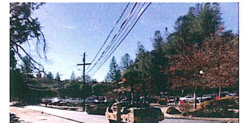
Paving on Mosquito Road
