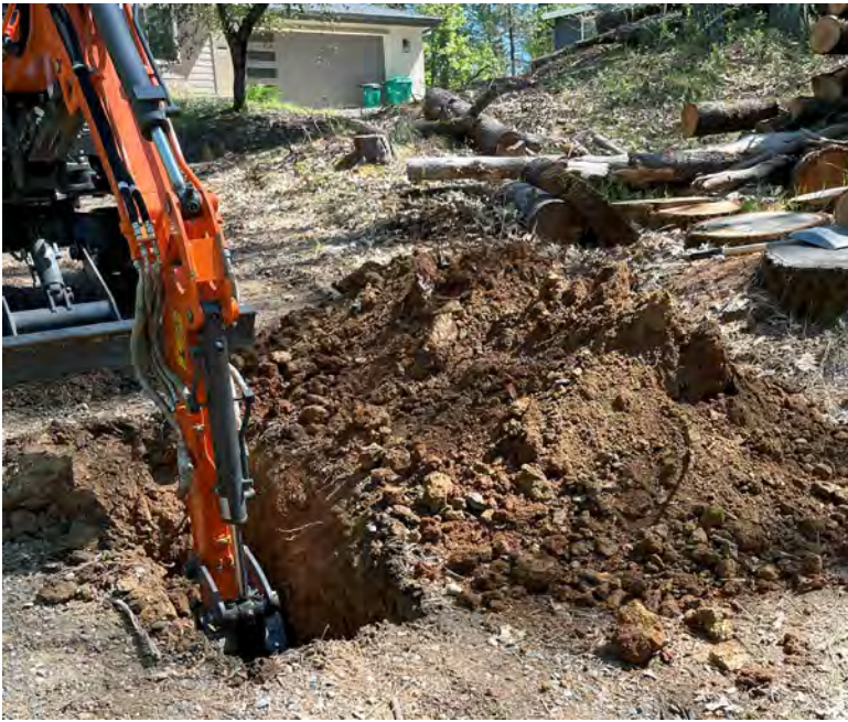
Photo #3: Test Pit TP3, looking north
