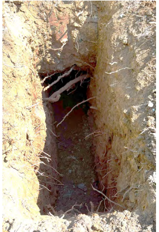
Photo #6: Test Pit TP1
