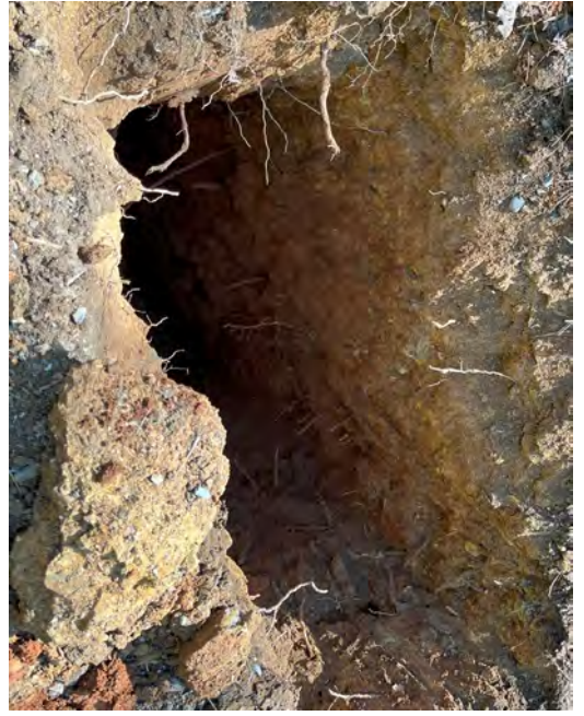
Photo #4: Test Pit TP4
