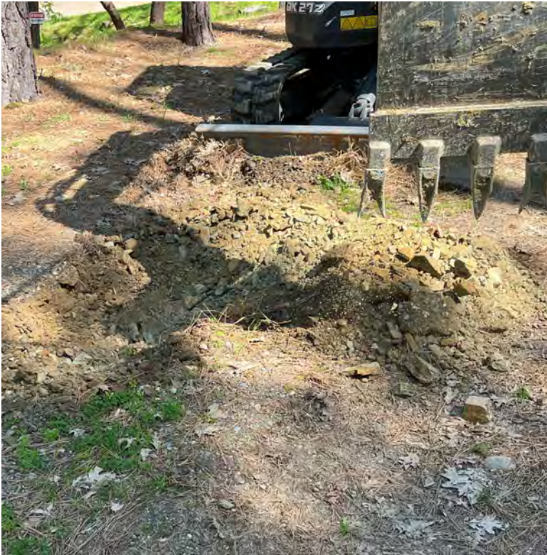
Photo #5: Test Pit TP2
