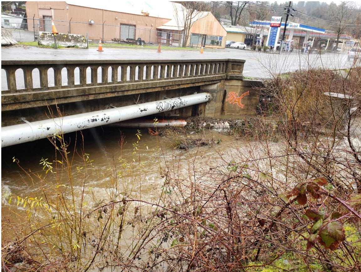
Photo 1. South Side of Existing Bridge (Looking East)
