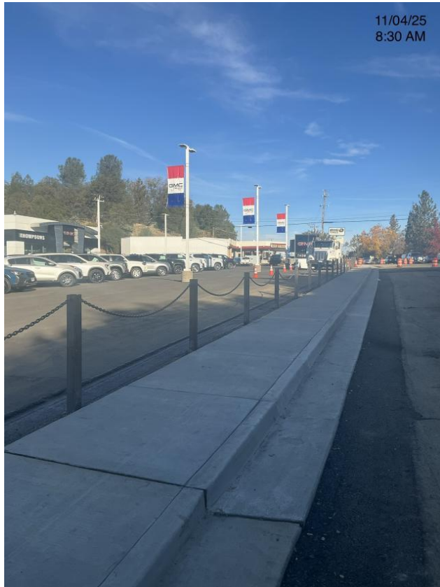
West Side Curb, Gutter Sidewalk
