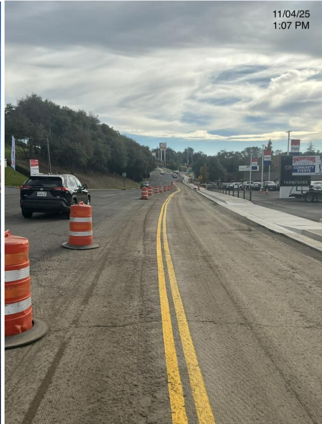
Preparation for traffic switch
