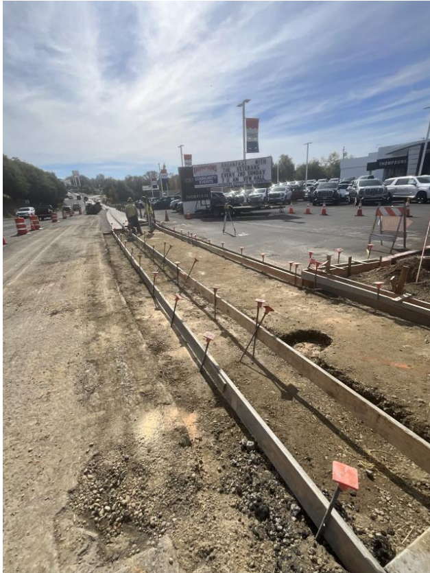
Forming driveways, curb, gutter, and sidewalk
