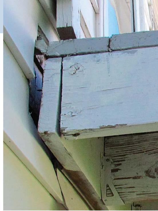
**Detaching ledger.** In this case, the homeowner noticed the failure of the nailed connection before the deck gave way. In other cases, decks have given way suddenly, often when they've been loaded with people.
