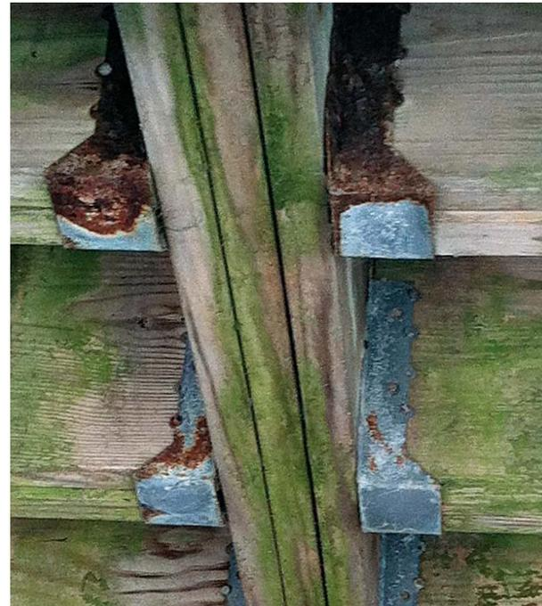
**Use the right joist hangers.** Although galvanized, the hangers on this seaside deck are rusty and nearing failure. Regular inspection of hardware is a good idea.
