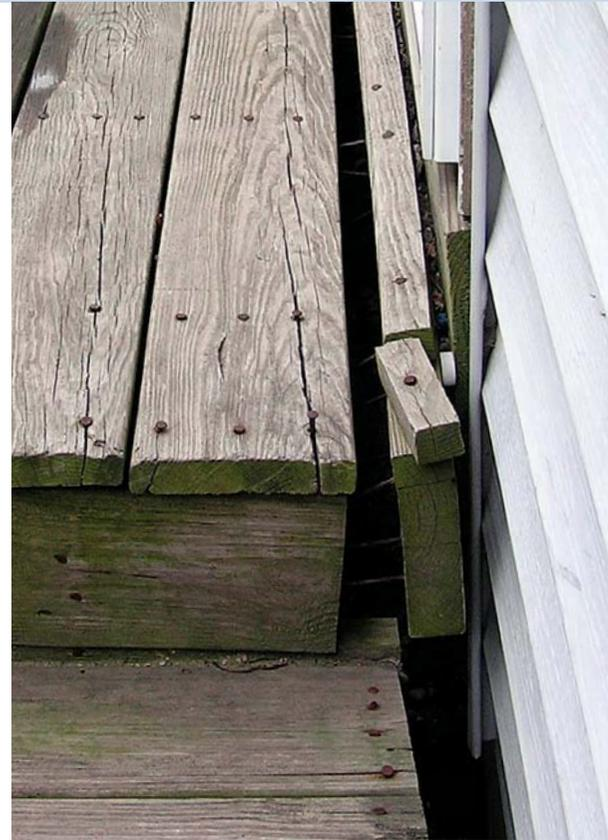
**Nails alone don't do the job.** This small deck was assembled by driving nails through the back of the ledger into the joists' end grain prior to installation. Toenailed joist-to-ledger connections are more common but also likely to fail.
