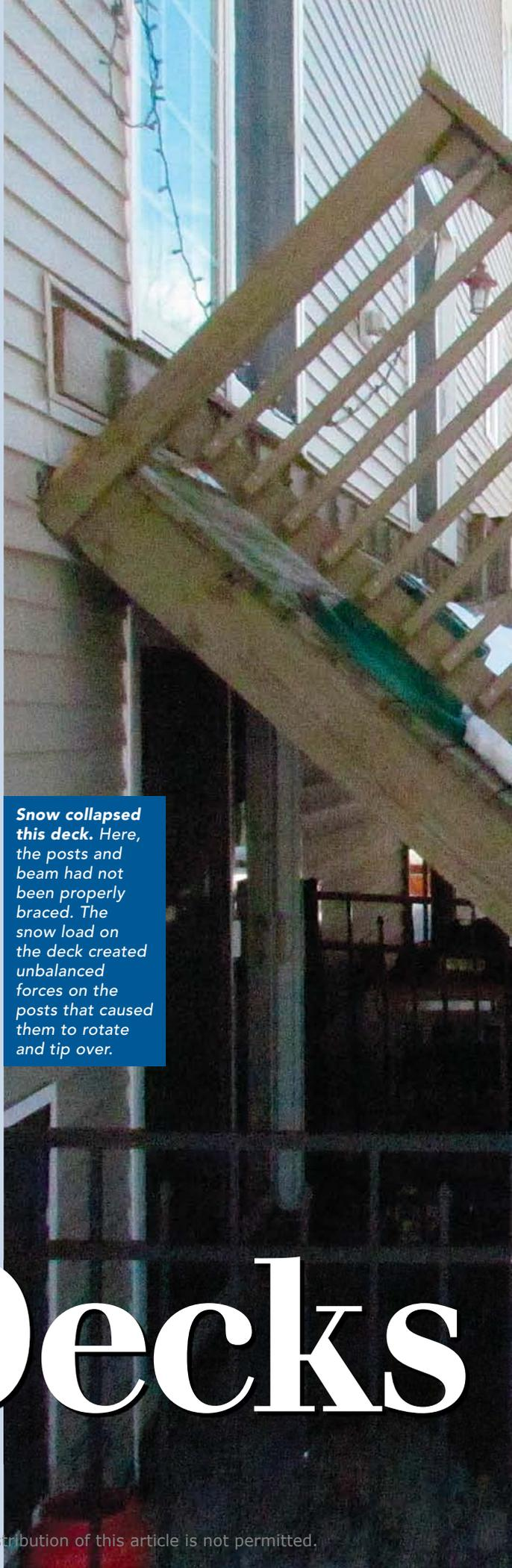
**Snow collapsed this deck.** Here, the posts and beam had not been properly braced. The snow load on the deck created unbalanced forces on the posts that caused them to rotate and tip over.
