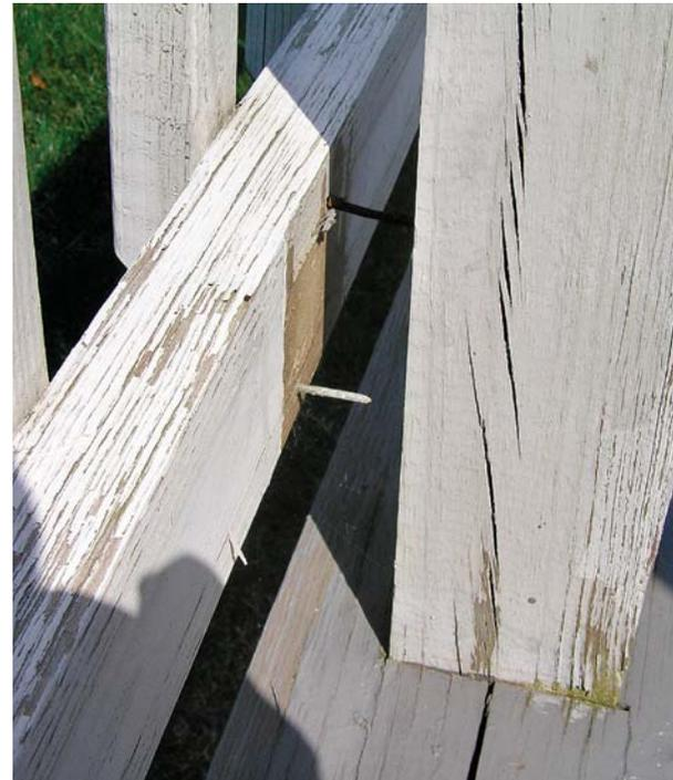
**Don't rely on nails.** This railing was just nailed to the outside of the posts. The nails eventually withdrew, and the railing pulled away.
