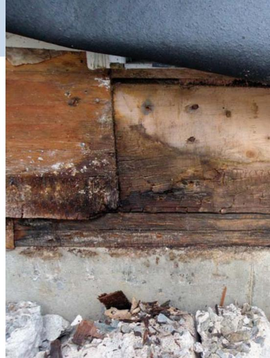
**Poor flashing leads to a rotted house.** Although this deck ledger had flashing, it was not properly integrated with the housewrap or building paper behind the siding. Water found its way to the house framing, rotting the rim joist and mudsill.
