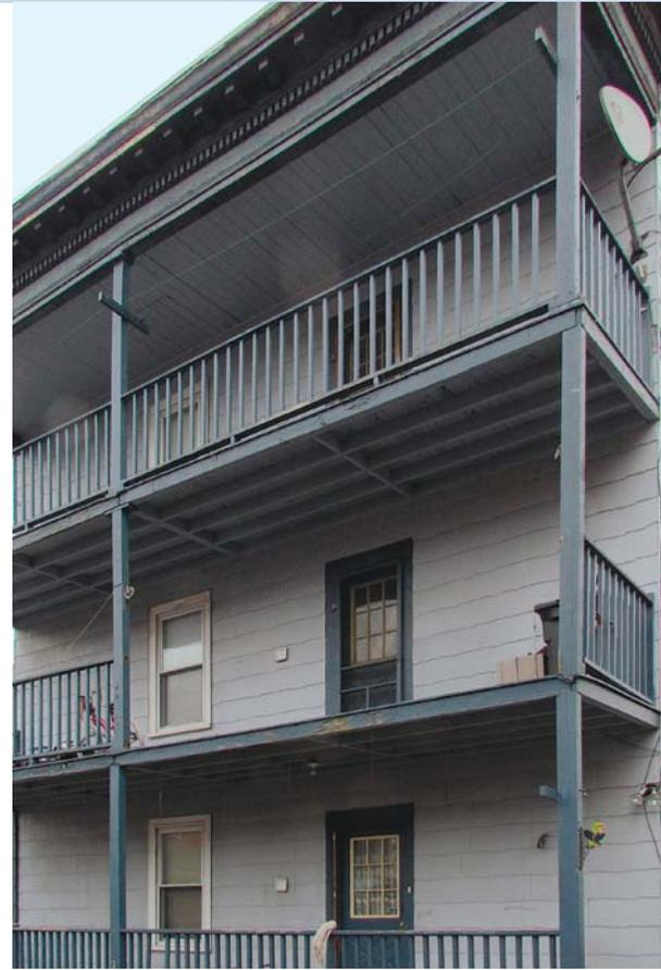
**Toenailed railing-to-post connection fails.** Over time, the wood decayed and the nails rusted. The weakened railing fell to the ground when someone leaned on it.
