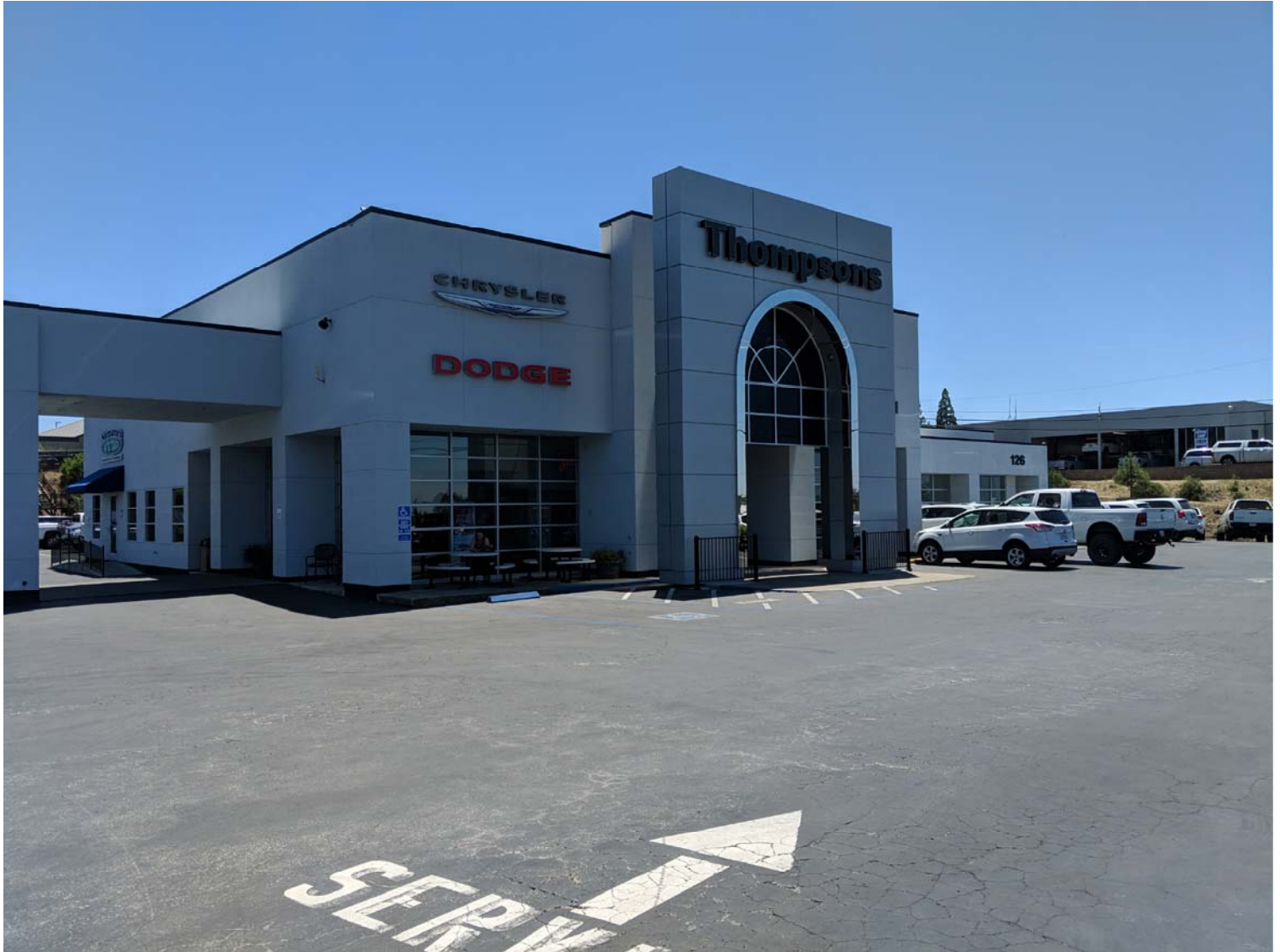
Exhibit B (View 1): Adjacent Commercial Property @ 126 Forni Rd
