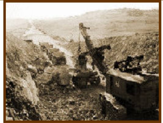
Construction of US 50 between Folsom and Placerville, March 1940
